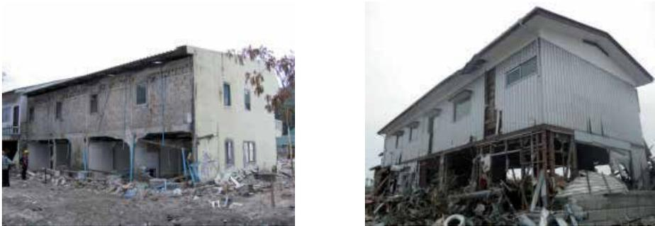
Fig. 25. Examples of building damage in the case of the 2004 Indian Ocean tsunami in Thailand and the 2011 Tohoku tsunami in Japan
