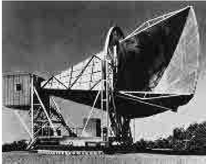
Radio waves thought to have originated in the primeval fireball that marked the start of the expansion of the universe were first detected by Arno Penzias and Robert Wilson with a sensitive receiver attached to this 15-m-long antenna at Holmdel, New Jersey.
